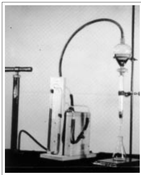
Figure 5. An apparatus to do flash chromatography in 1943. The photograph was supplied by C. David Gutsche, who did this work as part of his honors research.
